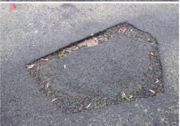
**Finding:** The surfacing is damaged creating trip points and **Action:** Repair damaged areas of surfacing exposing the concrete base
