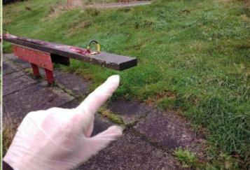
**Finding:** The ground clearance of the seats at the lowest point is less than 230mm and fails to meet the requirements of BS EN 1176 Part 6
