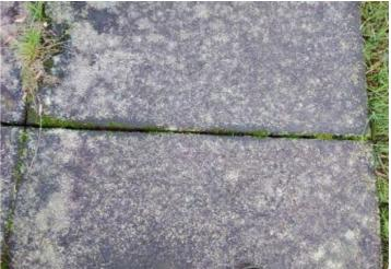
Finding: There are gaps opening in between the tiles on the Action: Monitor for any further deterioration and repair as tile surfaces around the site required
