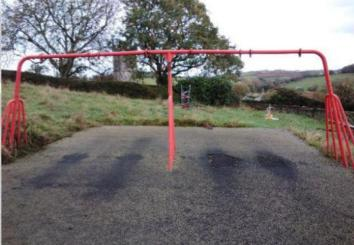
**Action:** Repair the frame defect and damaged wet pour safety surface prior to reinstating the missing seats and suspensions
