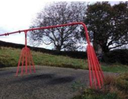
**Finding:** The seat(s) and suspension were missing at the time of inspection and the inspector was unable to make a full compliance assessment
