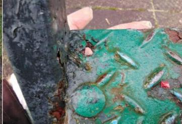
**Finding:** Parts of the steel on two steps have corroded excessively and the metal has perforated in places
