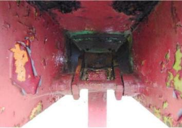
**Finding:** There is no gaiter protection for accessible moving **Action:** Monitor - No remedial work recommended parts (possible shear trap) as recommended in BS EN 1176
