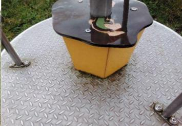
**Finding:** The bearing is showing signs of wear
